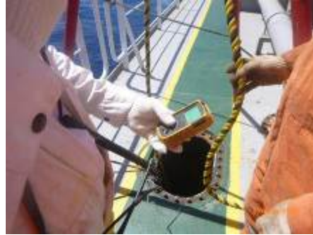
Oxygen and gas content inside the tank measured and found to be safe for entry
